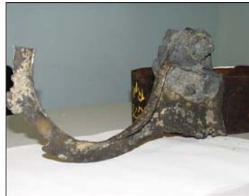
Corroded roof hanger.
